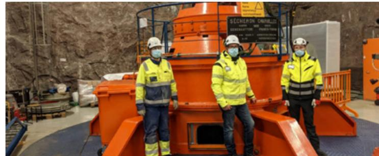
**We overhauled our Jumisko hydropower plant in Kemijärvi.** The overhaul increased the plant's capacity to produce balancing power and increased its power and energy efficiency.
