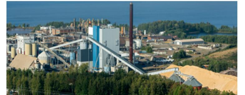
**Porin Prosessivoima decided to abandon the use of peat by the end of 2023.** Peat will be replaced by local wood-based fuel. We also decommissioned a separate coal boiler.
